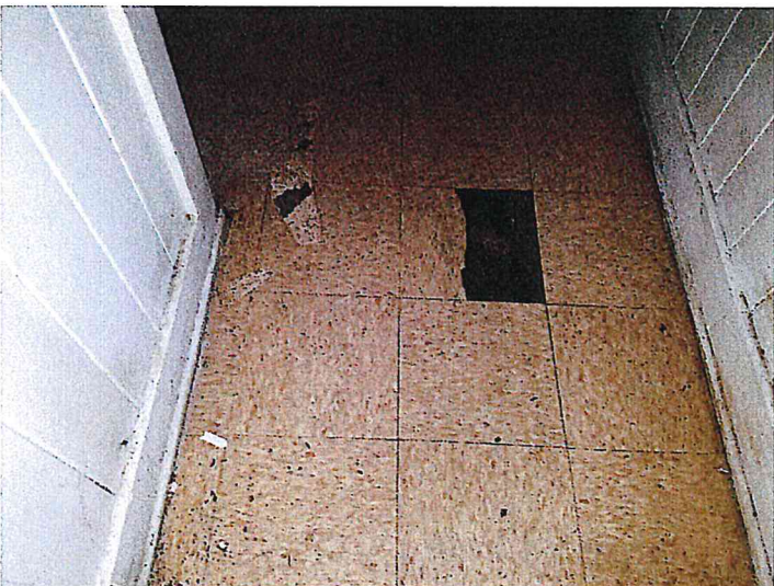
4/19/2016 SAMPLES S05 & S06 - 12X12 FLOOR TILE TAN PATTERN W/ BLACK ADH Pic (19).jpg
