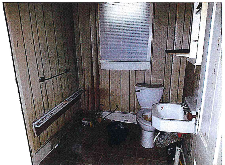
4/19/2016 513 A&B - INTERIOR B SIDE Pic (16).jpg
