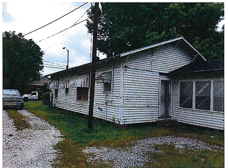
4/19/2016 EXTERIOR SIDE D - 513 A&B NE EVANGELINE THRUWAY Pic (04).jpg
