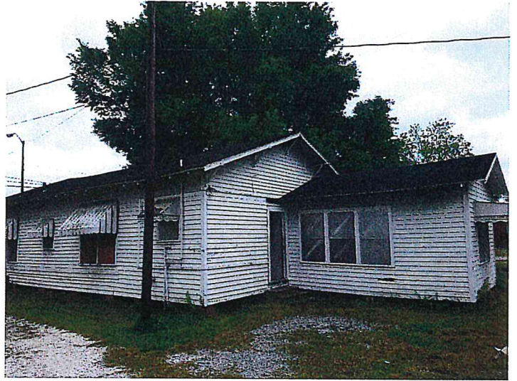
4/19/2016 SAMPLES S49 & S50 - SHINGLE ROOF & FELT MTRL Pic (22).jpg
